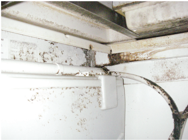
⌘ After a proper disinfection, this previously mold-/bacteria-fouled ice machine (inset) was fitted with a UVGI system.
